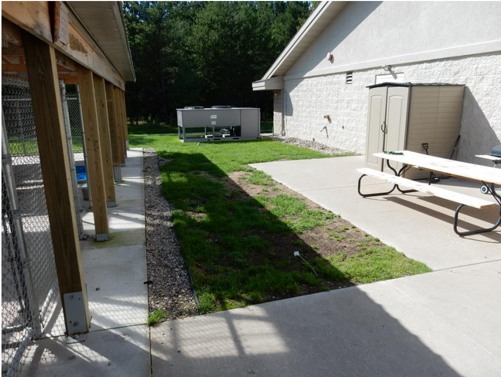
Before picture of area between building and outdoor runs.
