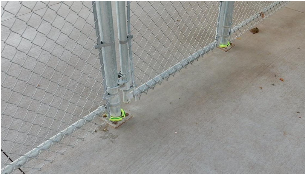
Fence modification to stop hoses from being damaged by mounting bolts
